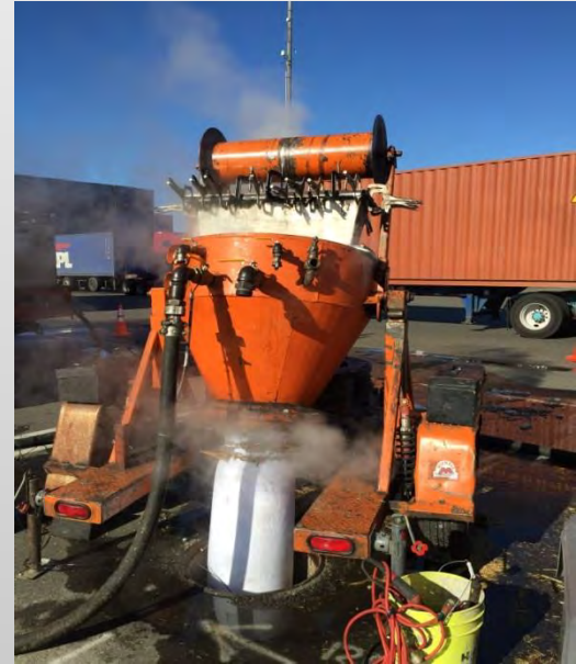
Cure-in-place pipe installation
