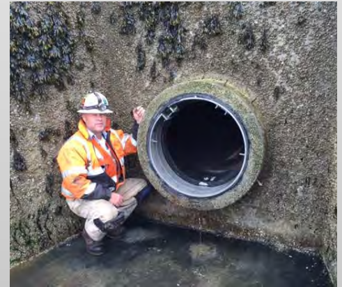
New tide gate installation
